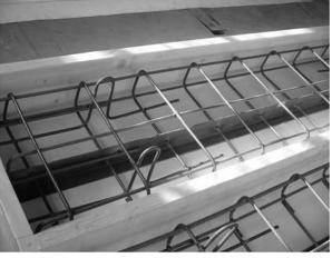
Figure 11 SPP beams and concrete reinforcement Slika 11. SPP grede i betonsko pojačanje
