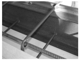
Figure 10 Preparation of SPC beams and the method of placing reinforcement bars Slika 10. Priprema SPC greda i metoda postavljanja profila za pojačanje
