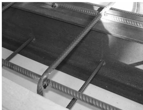
Figure 10 Preparation of SPC beams and the method of placing reinforcement bars
