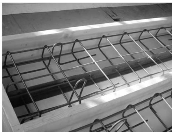
Figure 11 SPP beams and concrete reinforcement
