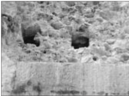
SL. 6. OSTATCI RUPA U KOJIMA SU SE NALAZILE NAJNIZIJE GREDE DRVENOGA MOSTA, KOJE NISU ODSJEČENE PA SU SLUZILE ZA SKELU KAMENOGA MOSTA, DESNA OBALA FIG. 6 REMAINS OF THE HOLES FOR THE LOWEST BEAMS OF THE WOODEN BRIDGE. THEY WERE NOT CUT OFF AND SERVED FOR THE SCAFFOLD OF THE STONE BRIDGE, RIGHT BANK
