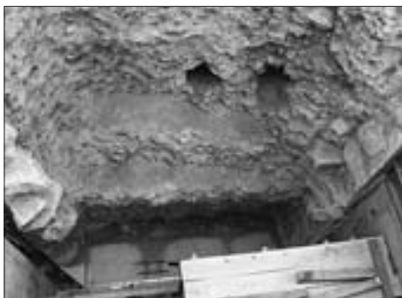
SL. 7. OSTATCI RUPA U KOJIMA SU SE NALAZILE NAJNIZIJE GREDE DRVENOGA MOSTA, KOJE NISU ODSJEČENE PA SU SLUZILE ZA SKELU KAMENOGA MOSTA, LIJEVA OBALA FIG. 7 REMAINS OF THE HOLES FOR THE LOWEST BEAMS OF THE WOODEN BRIDGE. THEY WERE NOT CUT OFF AND SERVED FOR THE SCAFFOLD OF THE STONE BRIDGE, LEFT BANK
