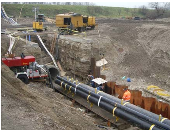
Fig. 2 Package of pipes in front of the tunnel
