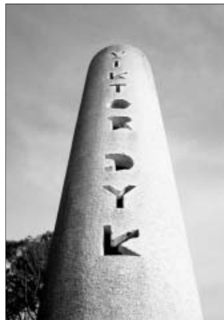
Sl. 19. SPOMENIK VIKTORU DYKU, DETALJ BETONSKOG MONOLITA Fig. 19 MONUMENT TO VIKTOR DYK, CONCRETE COLUMN, DETAIL
