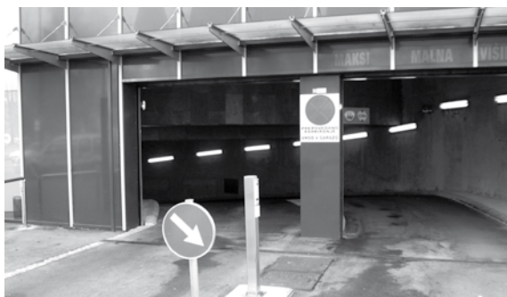
Figure 10. Underground car park entrance (Photo Courtesy of Ljubljana Fire Brigade)
