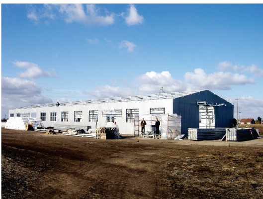
Figure 6 Wall and roof panels made with SSLC in profiled metal sheets
