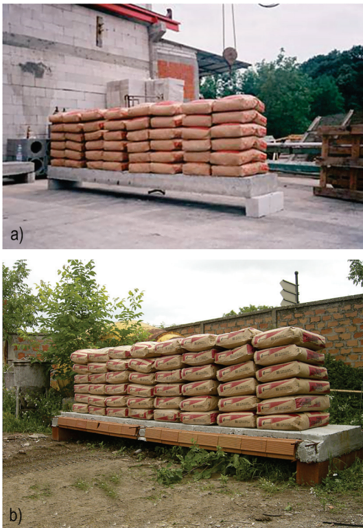
Figure 13 a) Testing of 4 m span reinforced concrete slab made with SSLC and b) an ordinary semi-precast FERT floor slab with the same span range
