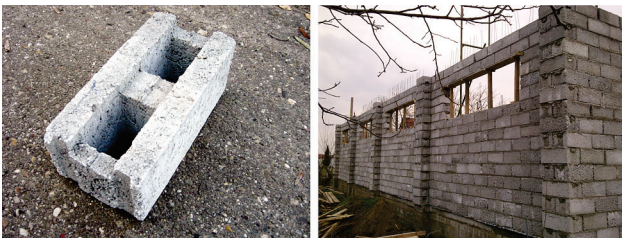
Figure 5 "Eco-keko" formwork - insulation hollow blocks for masonry made from SSLC (left) and a reinforced, core-filled concrete block structure made with these blocks
