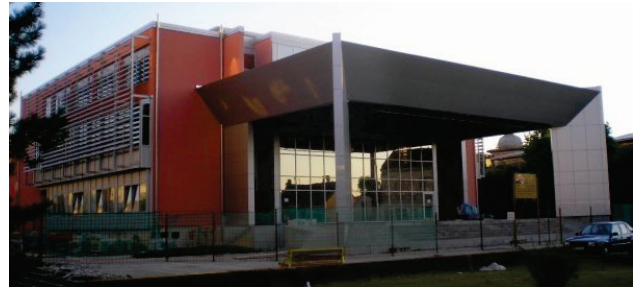
Figure 34 The appearance of the building facade after rehabilitation
