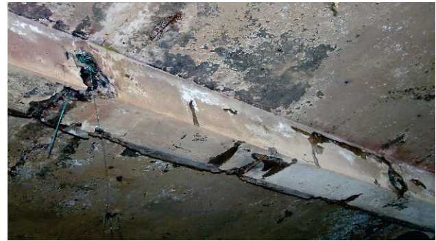
Figure 12 RC beam above the first floor (J-K/2)
