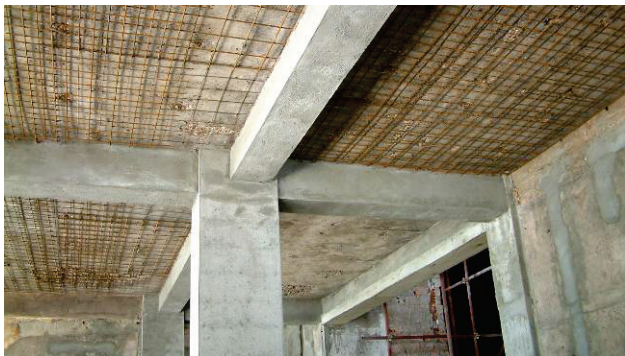
Figure 21 View of columns and beams after repair
