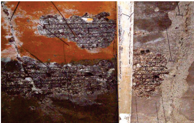
Figure 14 RC slab above the first floor (K-L-M/3-5)
