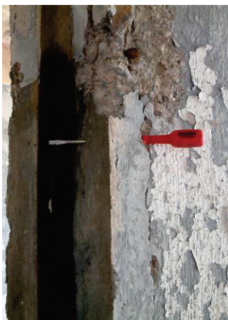
Figure 11 RC column K/2 (first floor)
