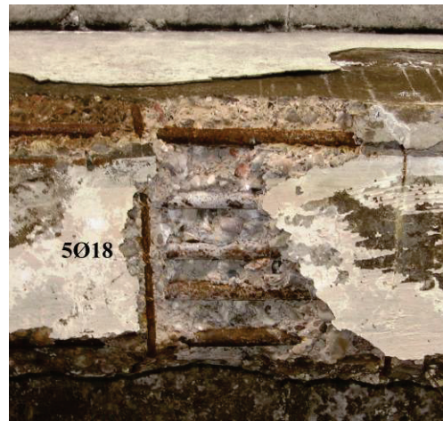
Figure 5 RC beam M/3-4' above the first floor
