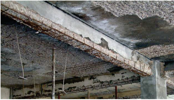
Figure 20 RC beam prepared for reparation
