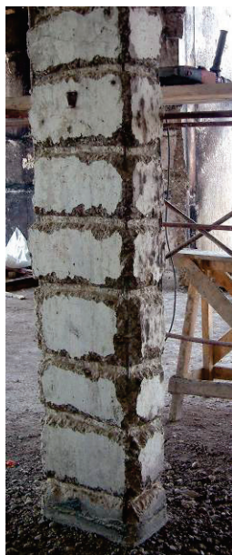
Figure 17 Preparing of RC columns for confinement
