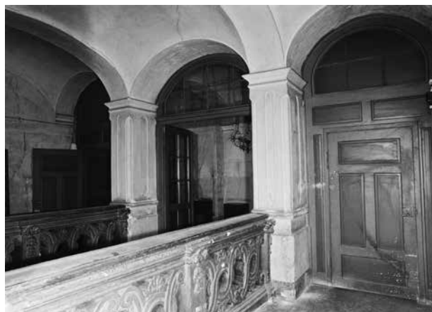
7. Stubište u prvom katu, pogled prema sjeverozapadu, 1985. (Arhiv HRZ) / Staircase on the first floor, northwest view, 1985 (Croatian Conservation Institute)
