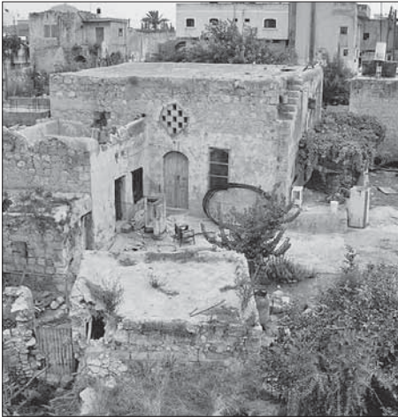
FIG. 11 FLAT ROOFING IN HOUSE SAID ABU HAMDEH IN ZEITA NEAR TULKARM
