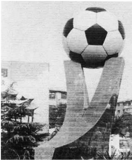
Figure 10 Hydrobulged steel football of 4000 mm diameter [10]
