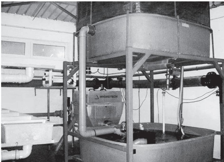
*Fig. 4. The mechanical and biological purifiers and the UV filter of the incubation unit work together to sustain good water quality in the hatchery*
