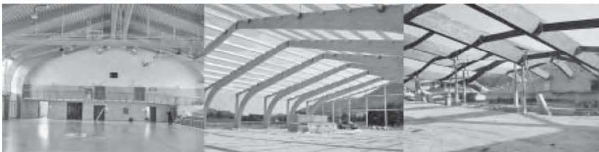
**Figure 8** Timber glulam construction (Hoja d.d., Škofljica, Slovenia)
