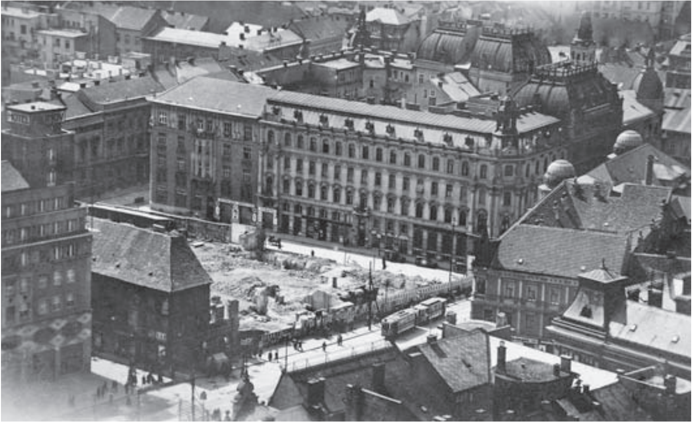
Sl. 1. Rušenje Zakladne bolnice, 1931. Fig. 1 DEMOLITION OF FOUNDATION HOSPITAL, 1931
