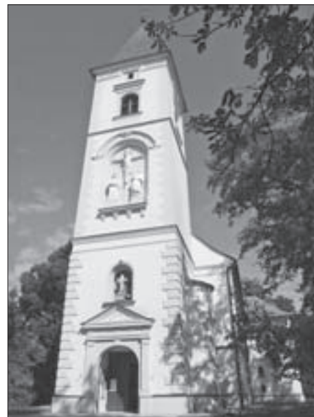
FIG. 18 MAIN FACADE OF THE PARISH CHURCH IN DUBRANEC, PRESENT STATE. CERTAIN DEVIATIONS FROM BOLLÉ'S DESIGN ARE DISCERNIBLE ONLY IN THE TOP OF THE Belfry WHICH NEVER RECEIVED THE ENVISAGED CLOCK.
