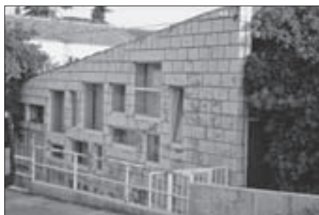
FIG. 10 NAUTICAL SCHOOL, DUBROVNIK: FENESTRATION OF THE WALLS, 1959
