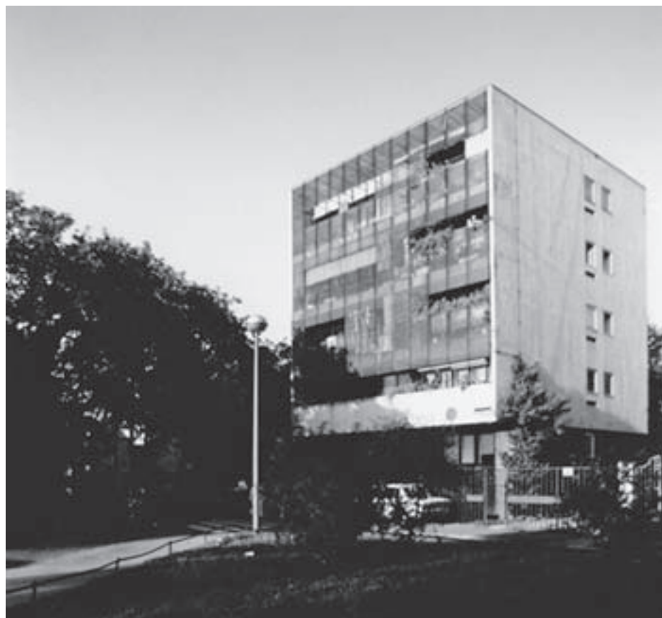
SL. 1. B. KRSTULOVIC: STAMBENA CETVEROKATNICA, PETRETICEV TRG 2, 1960., POGLED S JUGOZAPADA FIG. 1 B. KRSTULOVIC: RESIDENTIAL FOUR-STOREY BUILDING, 2 PETRETIC SQUARE, 1960, SOUTHWEST VIEW
