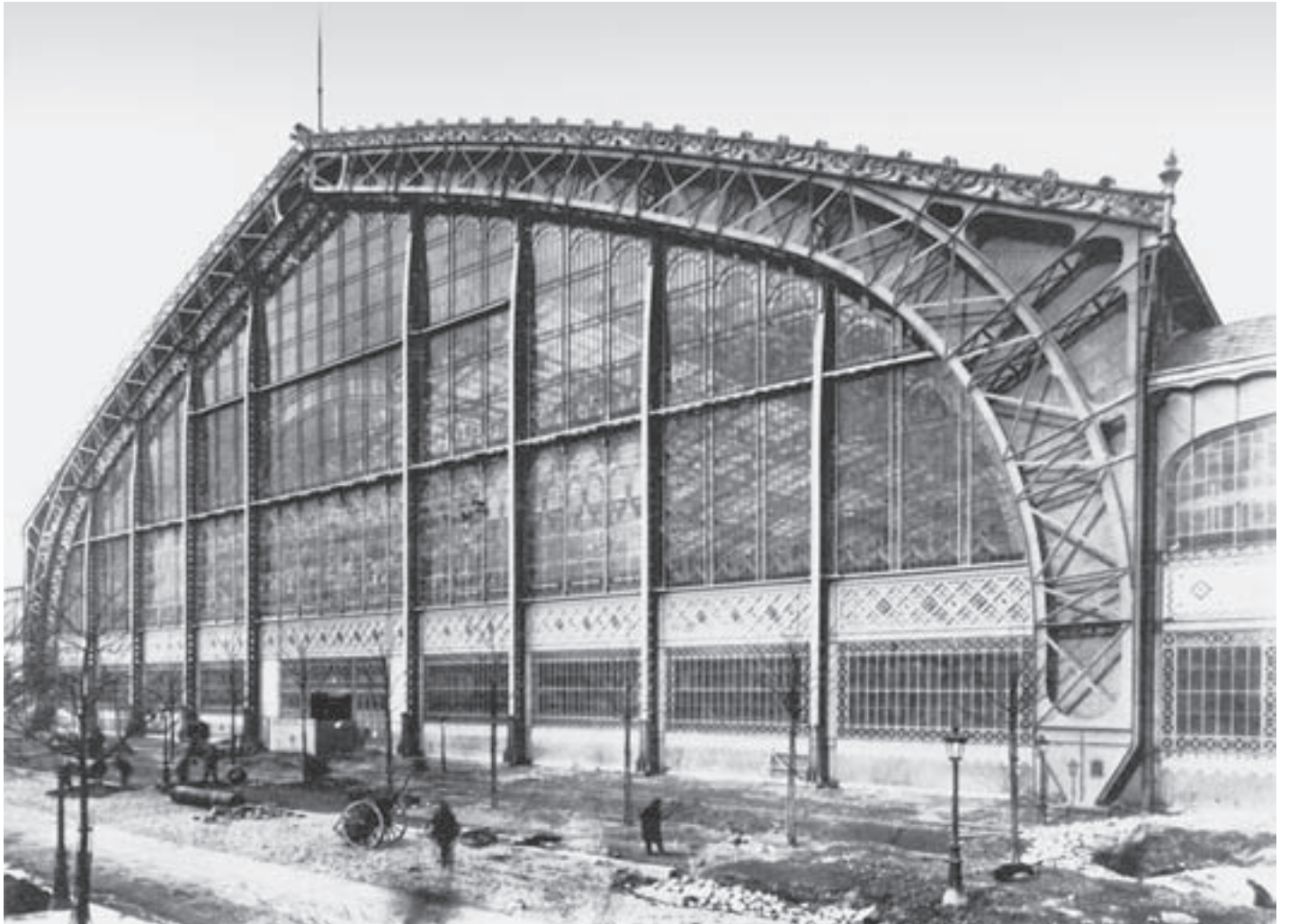
FIG. 1 GALLERY OF MACHINES: FIRST THREE-HINGED ARCH USED FOR A BUILDING STRUCTURE SL. 1. GALERIJA STROJEVA: PRVI PUTA KORISTEN TROZGLOBNI LUK U KONSTRUKCiji GRADEVINE
