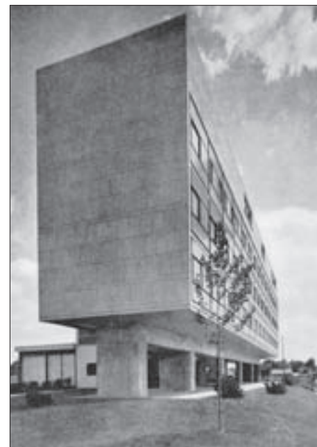
FIG. 9 LE CORBUSIER: SWISS PAVILION AT CITE UNIVERSITAIRE IN PARIS WITH A PASSAGE IN THE GROUND FLOOR AS AN EXAMPLE OF A POTENTIAL SOFT STOREY BUILDING
