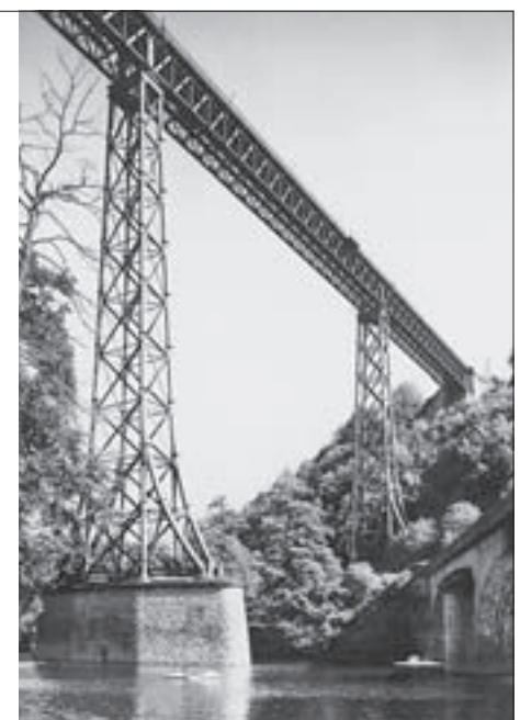
FIG. 6 GUSTAVE EIFFEL: A TOWER OF 300 METRES AND THE SUPPORTING PYLONS OF THE VIADUCT – THE BASIC SHAPE OF THE TOWER
