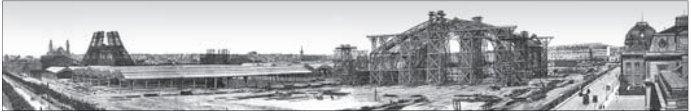
FIG. 5 GALLERY OF MACHINES DURING ERECTION, BEHIND IT THE ERECTION OF THE EIFFEL TOWER CAN BE SEEN
