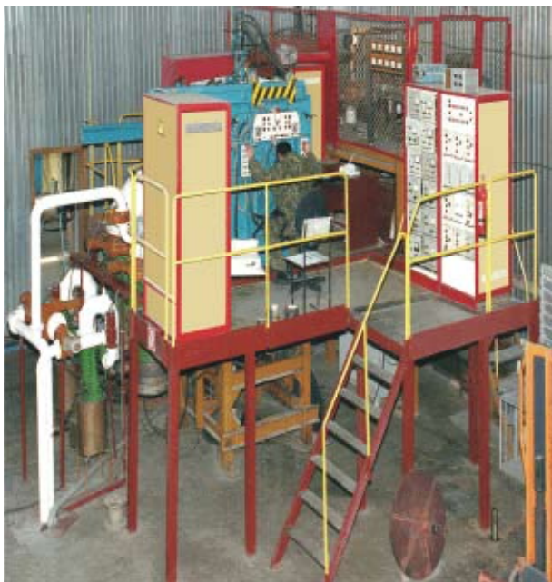
Figure 1. Surface appearance of industrial electron-beam facility UE-189
