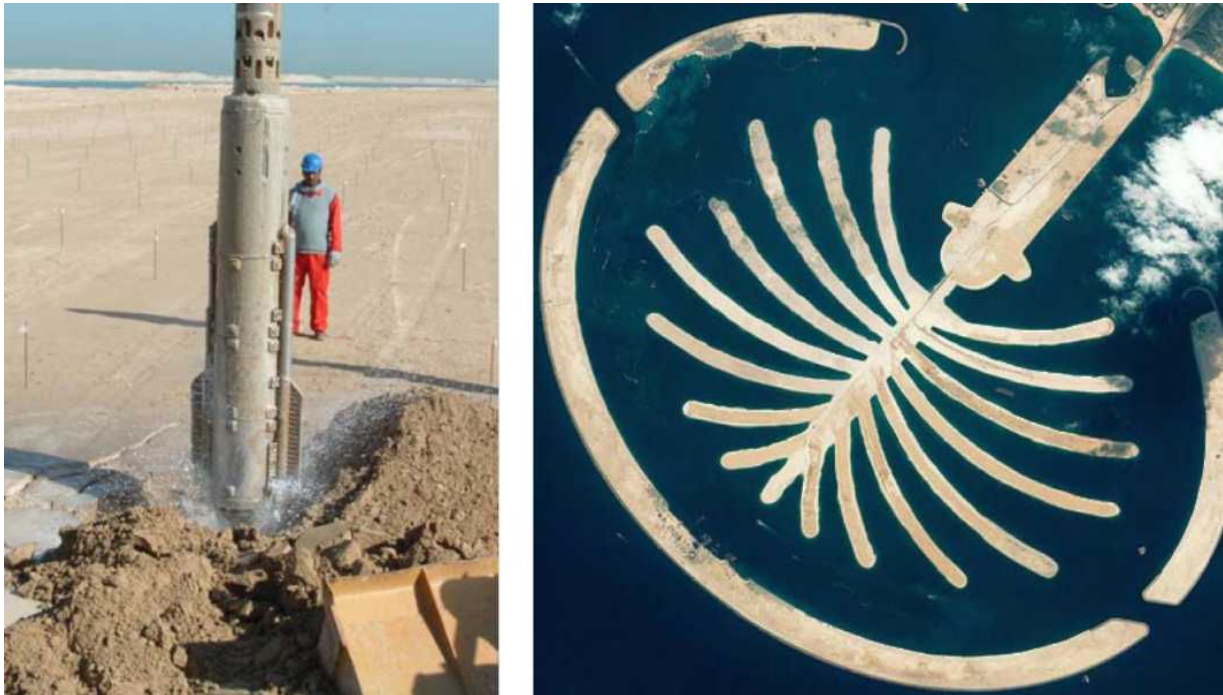
Figure 13 - Example for the contribution of geotechnical engineering to land reclaiming (Dubai)
