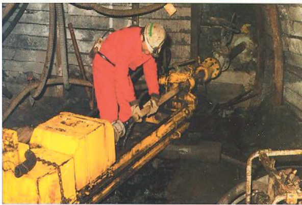
Figure 3 Degasification borehole drilling
