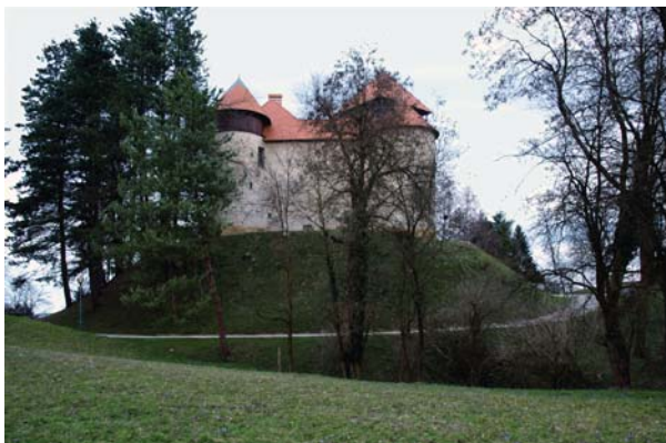
Slika 2. Pogled s jugozapada (snimio: Z. Čučković). Figure 2. View from the south-west (photograph by: Z. Čučković).
