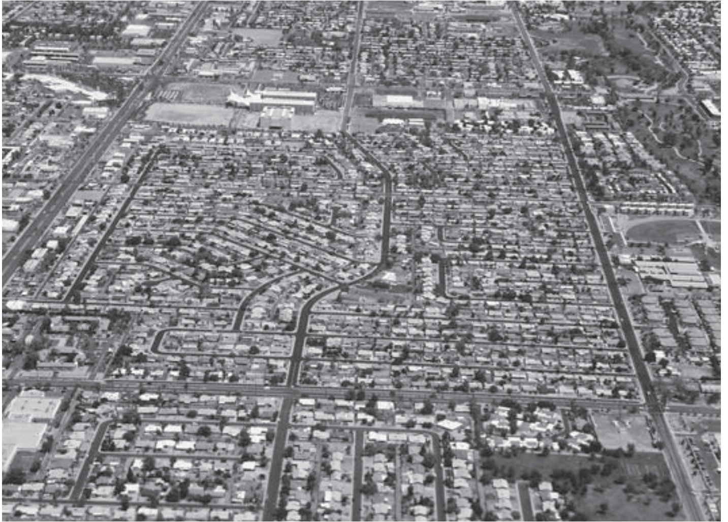
FIG. 1 VIEW UPON ONE OF MANY US CITIES BUILT ACCORDING TO LAND ORDINANCE ACT OF 1785 SL. 1. POGLED NA JEDAN OD MNOGIH GRADOVA IZGRADENIH PREMA LAND ORDINANCE ACT IZ 1785.
