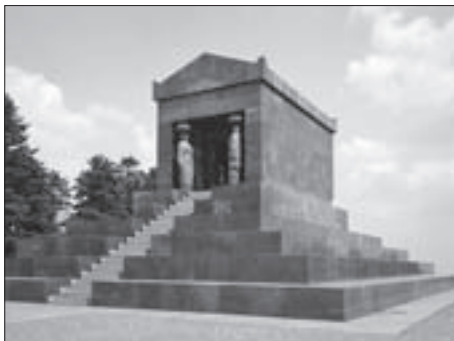
SL. 14. I. MESTROVIC: SPOMENIK NEZNANOM JUNAKU, AVALA KOD BEOGRADA, 1937. FIG. 14 I. MESTROVIC: MONUMENT TO THE UNKNOWN HERO, AVALA NEAR BELGRADE, 1937
