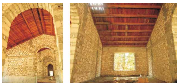
Fig. 5. and 6. The photographs taken in September 2003, showing the interior of one of the abandoned buildings, provide insight into the original project and the condition of the buildings at the time the construction was stopped. Spacious axially symmetric rooms, high ceilings, space filled with daylight, large windows placed considerably low, open wooden roofs and a central corridor with arches set into transversal bearing walls enclose a simple interior of striking aesthetics that can hardly be related to the notion of a place of torment or punishment. This building was completely renovated for the hospital's needs in 2005 when the interiors in the photograph were open for creative, occupational and recreational therapy, with minimal interventions employed. Compare Figures 10 & 11. Photo by I. Juretić.
