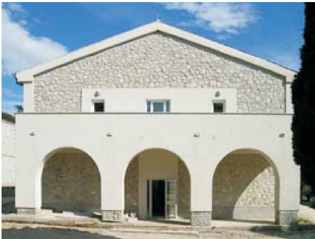
Fig. 9. The facade of one of the reconstructed two-story buildings in August 2005. By giving prominence to the existing qualities, restraining the contrasts between light and dark, and compensating for the drawbacks, the subtle renovation emphasised the scope of the original architectural idea. Photo by I. Juretić.
