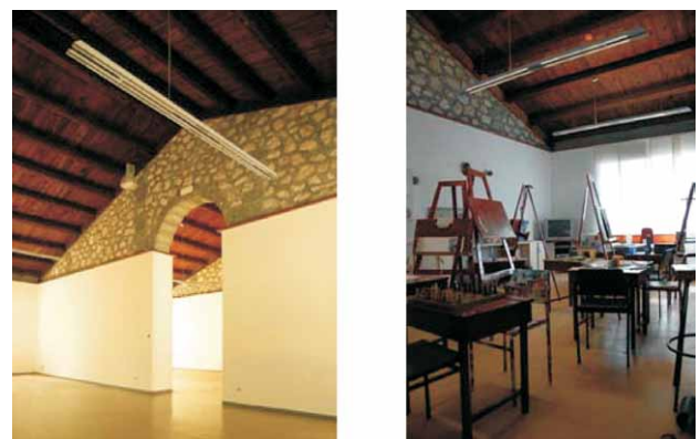
Fig. 10. and 11. Rooms for creative, occupational and recreational therapy on the first floor of the building after the reconstruction. Compare Figures 5 & 6. Minimal interventions on the building have emphasised most of its existing qualities and have had an extraordinary effect. The dilapidated rooms of one of the old buildings were turned into a modern, spacious and cheerful hospital facility intended for creative and recreation therapy. Photo by I. Juretić.
