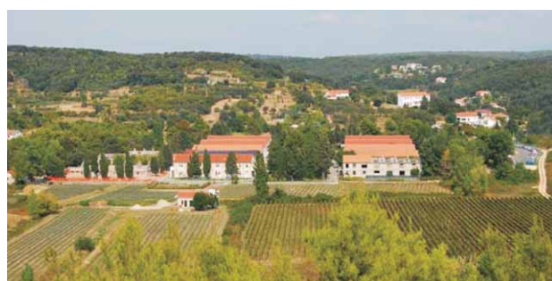
Fig. 8. The hospital complex in the photograph taken in September 2009 from a nearby hill, once the location of a quarry opened for the buildings' construction. The field of Kapor is planted with vineyards, the hospital agricultural land is covered in lavender and the grounds are dominated by the tall stone pines, cypresses and sycamores that have adorned the surroundings of the existing buildings almost since their construction, although they have grown to exceed them in height. Photo by I. Juretić.
