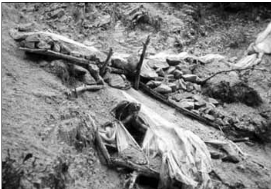
Fig. 7 Barrier in a dolomite erosion gully Sl. 7. Prepreka u jaruzi oblikovanoj u dolomitu
