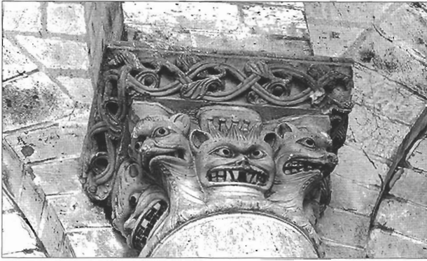
Fig. 12. Church of Notre Dame in Cunault, capital in the choir (foto: M. Vicelja)
