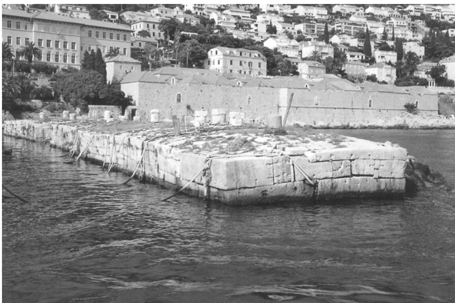
Slika 10. Valobran Kaše i Lazareti Figure 10. Seawall Kaše and Lazareti
