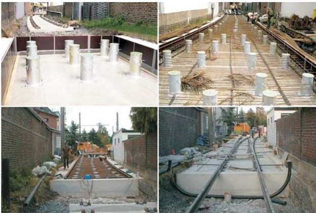
Figure 16 Floating slab track on springs
