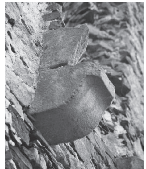
FIG. 3. GARIĆ BURG, NORTH-FACING DEFENSE TOWER, CANTILEVER OF THE LAVATORY, SECOND FLOOR
