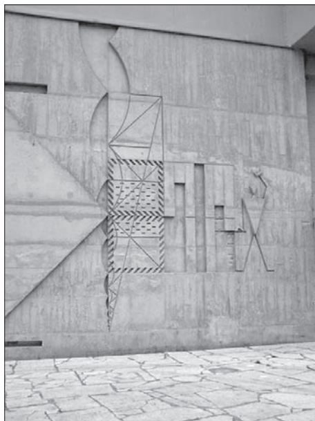
SL. 9. RELJEF NA ZIDU PRIZEMLJA UNITÉA U BRIEY-EN-FORÊTU FIG. 9. RELIEF ON THE WALL OF THE GROUND-FLOOR LEVEL, THE UNITÉ IN BRIEY-EN-FORÊT
