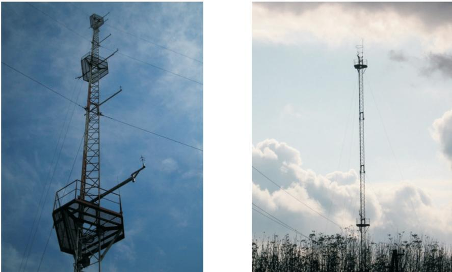
**Figure 2.** Closer (*left*) and distant (*right*) view of the mast. Ultrasonic anemometers are mounted at 12, 20, 32, 40, 55 and 62 m a.g.l.
