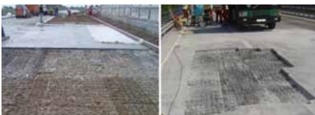
Figure 1. Replacement of existing layers during deck slab repair on bridges
