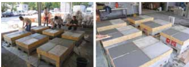
Figure 7. Reshaping concrete freshly placed onto the surface of all 6 blocks
