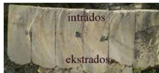
Figure 4. A remaining part of the original bridge's stone arch at spring, with a thickening above extrados
