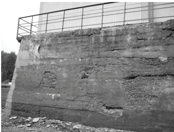
Figure 3 Appearance of concrete on the exterior of the shaft
