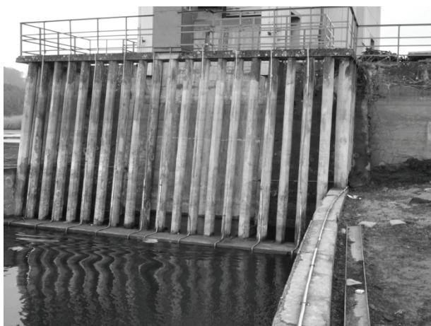
Figure 4 Appearance of protective grille
