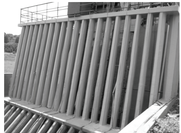
Figure 8 Appearance of protective grille after restoration
