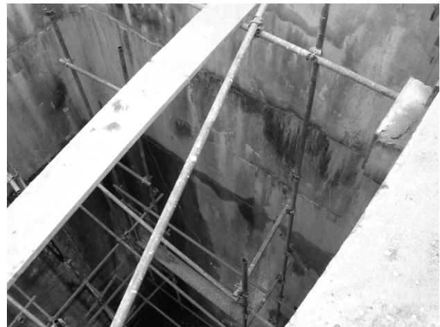
Figure 2 Concrete shaft within the structure
