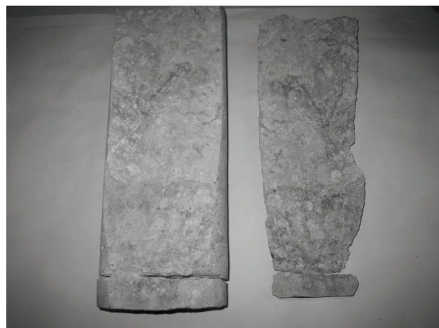
Figure 6 Appearance of the cylinder sample taken at the location of concreting joint
