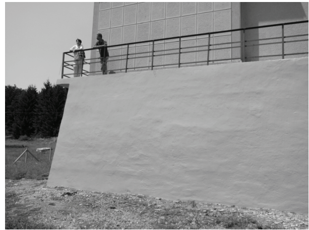
Figure 7 Appearance of the exterior concrete surface after restoration
