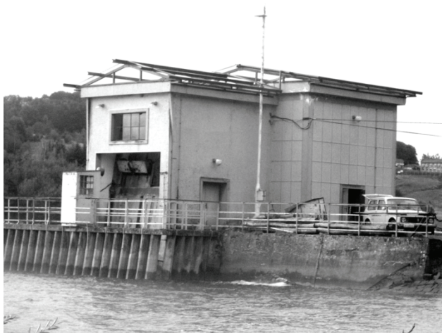
Figure 1 Appearance of the entry structure of "Vrta" HE
