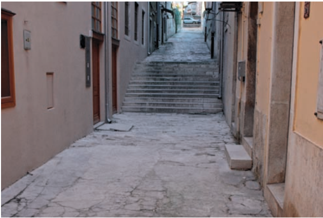
Sl.2a Pogled na donji dio Uspona Frana Glavinića prije novijih građevinskih i arheoloških radova 2011. godine (foto R. Zlatunić) Fig. 2a A view of the lower section of the Fran Glavinić Gradient, before the start of the more recent construction works and archaeological explorations in 2011 (photography R. Zlatunić).
