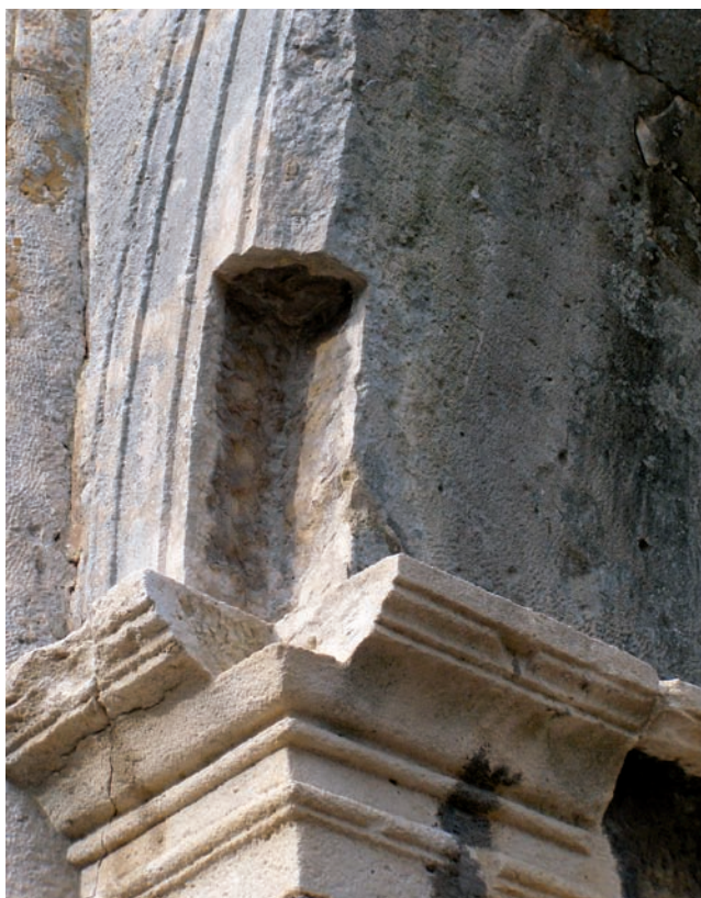
Sl. 4 Detalj pozicije odstranjenih kamenih nadogradnji. Fig. 4 A detail showing the position of subsequent stone additions that were removed.
