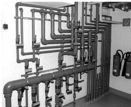
Slika 2. Razdjelnik sanitarne vode od PP-R 80 [1] Figure 2. Distributor of sanitary water made of PP-R 80 [1]
