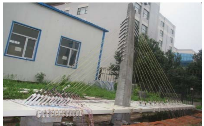
Figure 12. A constructed FRP bridge
