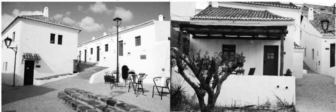
Figure 3 Aldeia da Pedralva after rebuilding
