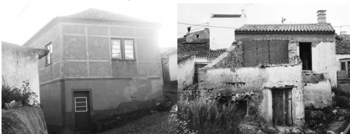
Figure 2 Aldeia da Pedralva before rebuilding
