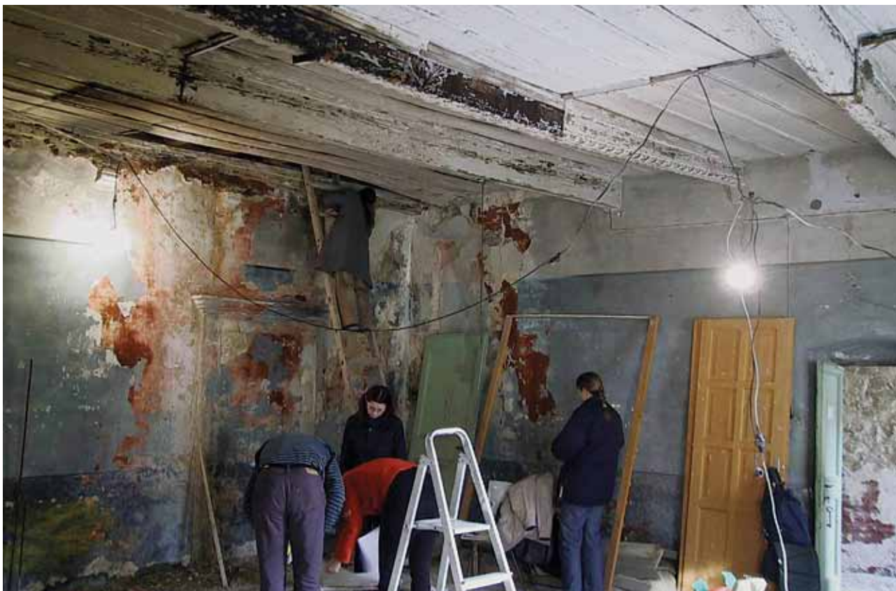
24 Interijer kuće prije radova sanacije i rekonstrukcije (foto: Giuseppe Sava, 2003.) Interior of the house prior to rehabilitation and reconstruction works (photo by Giuseppe Sava, 2003)
