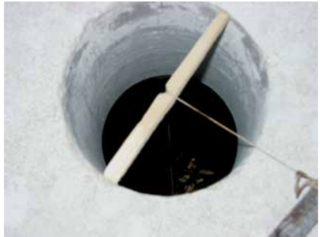
21 Centriranje položaja osovine mlinskog postrojenja (foto: Sanja Buble, 2008.) Centering the position of the axle of the mill mechanism (photo by Sanja Buble, 2008)
