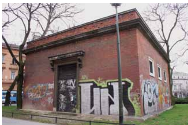
Transformatorska stanica na Rooseveltovu trgu, 2010. godine (Fototeka GZZSKP-a) Substation on Roosevelt Square, 2010 (Photo archives of GZZSKP)
