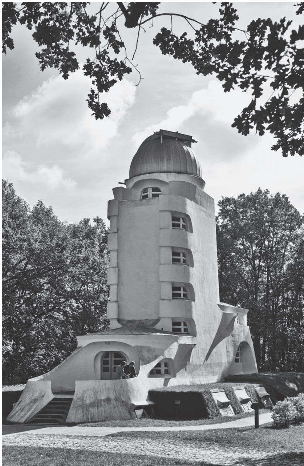
FIG. 1. ERICH MENDELSON, THE EINSTEINTURM (EINSTEIN TOWER), CONCEPT 1917, BUILT 1919-1921, POTSDAM SL. 1. ERICH MENDELSON, EINSTEINOV TORANJ, KONCEPT 1917., IZGRADNJA 1919.-1921., POTSDAM
