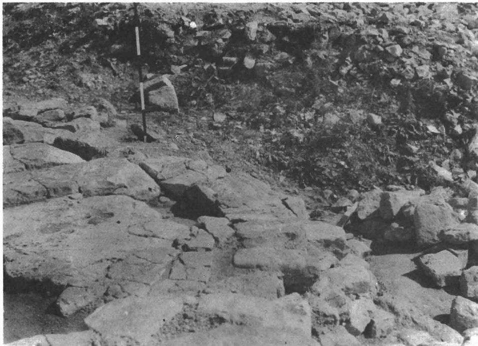
Sl. 7. Kašić, Mastirine. Temeljni ostaci jugoistočne (III) apside prije rekonstrukcije. — Kašić, Mastirine, Remains of Foundations of south-east (III) apse before reconstruction
