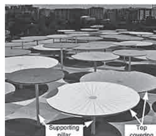
Figure 1 Schematic representation of an „urban forest“ with parasol elements (the supporting pillar and the top covering)
