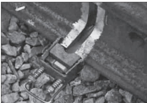
Figure 5 Ceramic backing with metal insert
