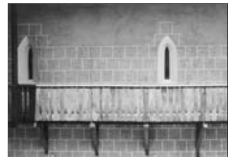
FIG. 23 ĐURĐEVAC CASTLE, GALLERY IN THE INTERIOR OF THE CASTLE AFTER RENOVATION
