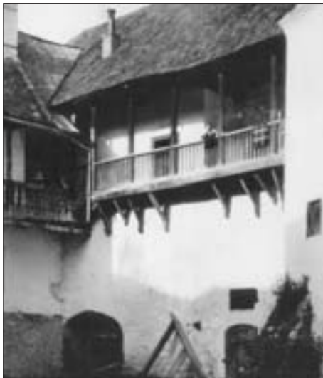
SL. 34. BURG ĐURĐEVAC, DVORIŠTE BURGA PO UPRAVO DOKRŠENOJ OBNOVI FIG. 34 ĐURĐEVAC CASTLE, COURTYARD IMMEDIATELY AFTER RENOVATION
