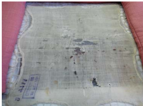
7.29 Konzervatorsko-restauratorski radovi Conservative-restorative procedure
