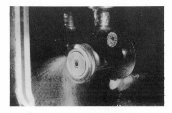
Fig. 5. Milling of the ceramic block in the chamber seen in Fig. 1 on the unit's lower left.
